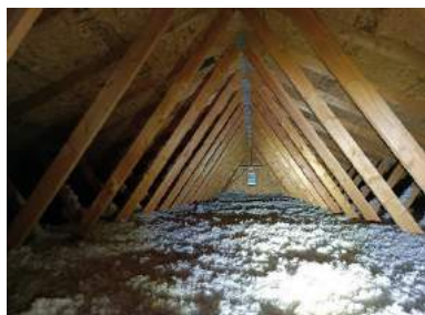
Example: Attic framing / insulation
